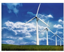
ENERGETICO ENERGY INDUSTRY
